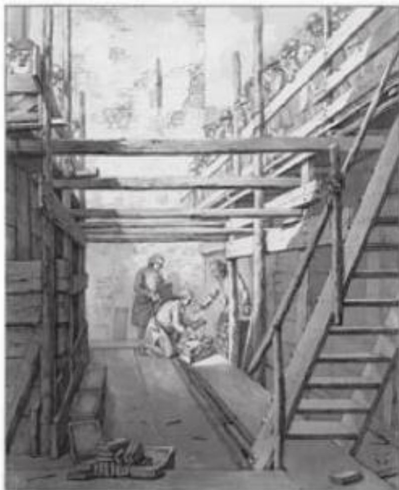
The ceremony of laying the foundation stone of the Felix Meritis Building on 23 June 1787 by Cornelis Sebille Roos. Drawing by C.L. Hansen.
